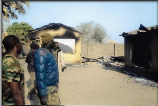
PIC: Nigerian Army Officers looking at some burnt buildings at Kunini in Lau Local Government Area.
